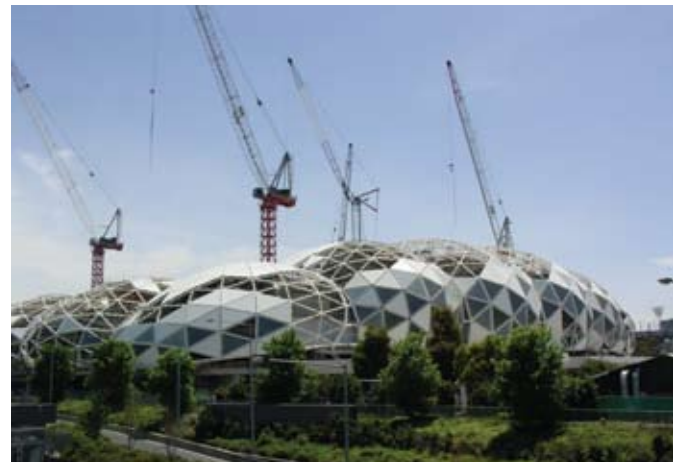
Melbourne's Rectangular Stadium under construction. The geodesic dome design uses only 50% of the steel in a typical stadium roof
